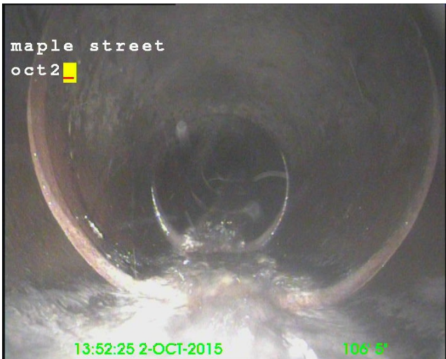
A clean sewer pipe with flow
